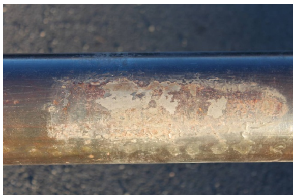
Pic # 3. Surface rust
